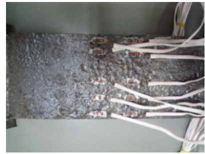
(c) Local corrosion type (F-10)
