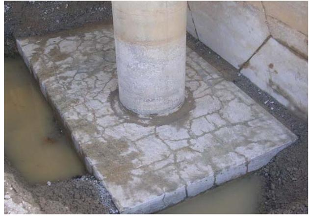
Figure 1 Map cracking in a pile cap
