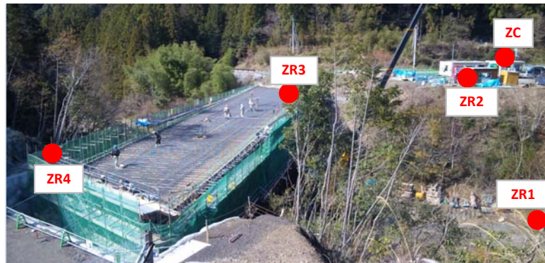
Figure 6 ZigBee Coordinator and Reuters on construction site
