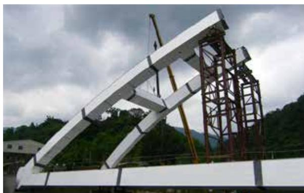
Fig. 15 The Bridge hosting work
