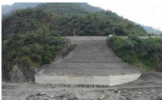
Fig. 14 The River bank protection works
