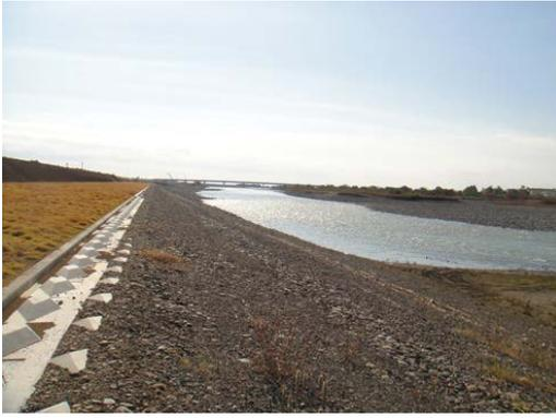
**Figure 5** River bank erosion protection and river terrace
