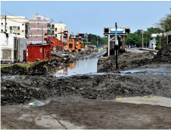
(Fig. 7) The height of deposited soil in Linbian Railway Station was almost as high as the platform.
