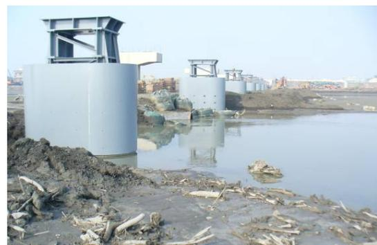
(Fig. 13) Adding 2 M high formed steel structure on top of pier and the RC piers are clad with steel plate and constrained with concrete.
