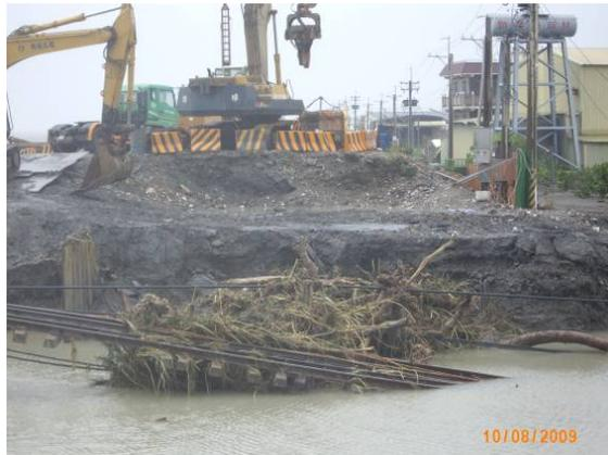
(Fig.10) Damages to north abutment 、Washed off Road Base.
