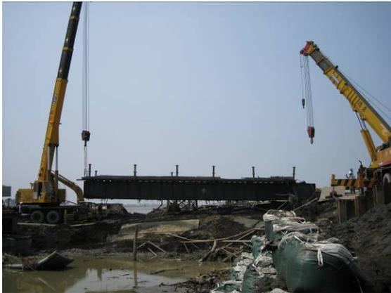
(Fig. 11) Bridge Steel Beams are totally lifted and moved away from site
