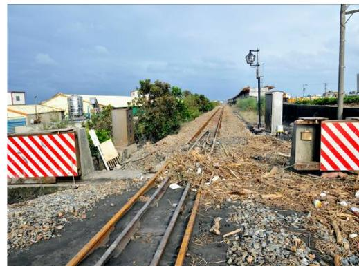
(Fig. 16) South side gate was intact after the disaster due to deposit and stacking of drifting articles brought by the flood.
