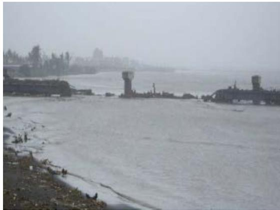
(Fig. 9) Washed off 2 piers and 3 spans (P10/11/12)
