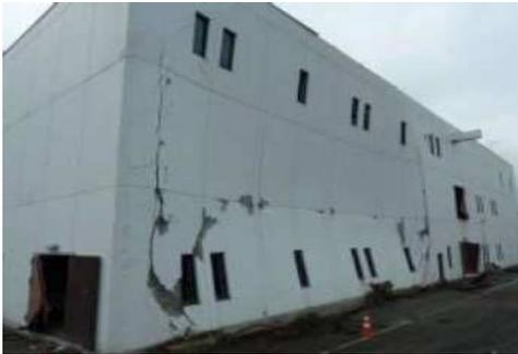
Figure 3: Damage of RC wall in Sendai, Miyagi
