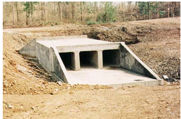
Fig.5b Concrete box culvert
