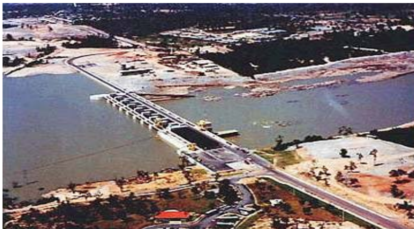
Fig.8 Pak Mool dam in Ubol Rachathani constructed using roller-compacted concrete with fly ash content of 68% of the total cementitious materials.
