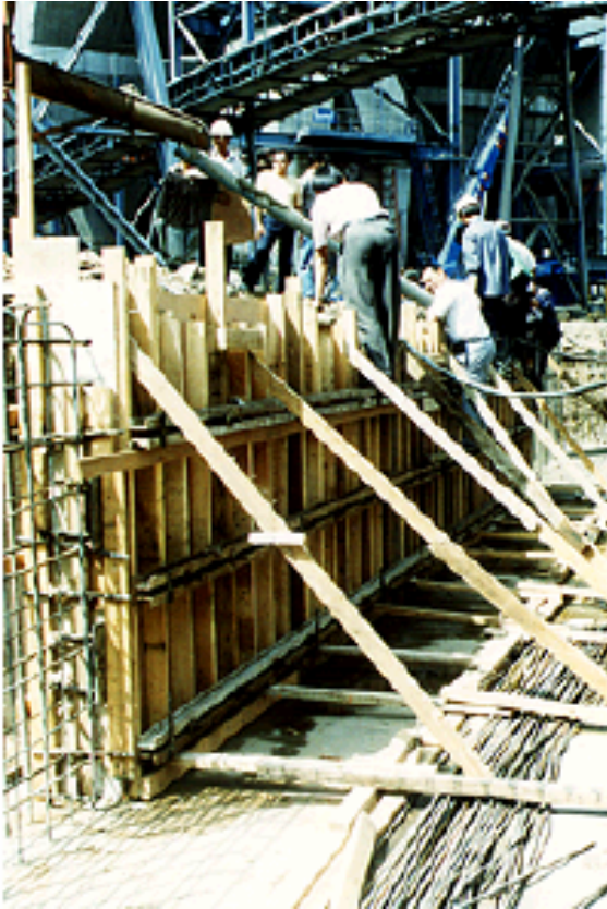
Fig.5a Concrete wall
