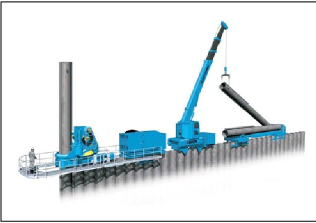
Figure-1. The Press-in Method
