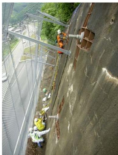
Picture 4. The investigation by new type of the hydraulic jacks
