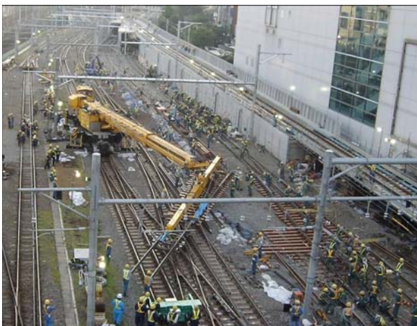
Figure 4 Scene of rail switchover (1)
