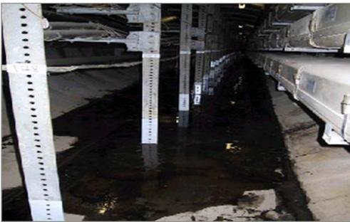
Figure 10 Inflow of groundwater into the tunnel
