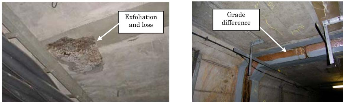
Figure 4 Example of tunnel at abnormal state
