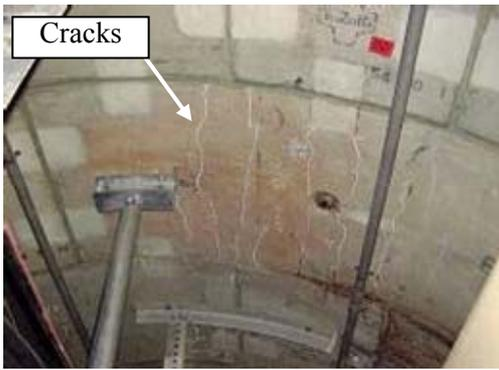
Figure 9 Cracks on the segments
