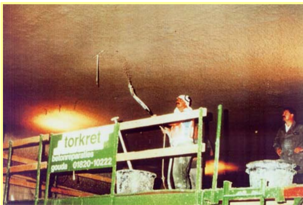
Figure 5.2 Mitigation measures by sprayed fire protection 6)
