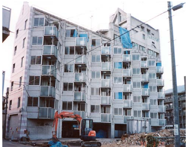
(a) Full view of the building (RC frame structure)
