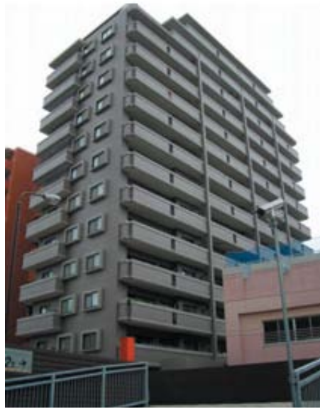
(a) Full view of the Building
