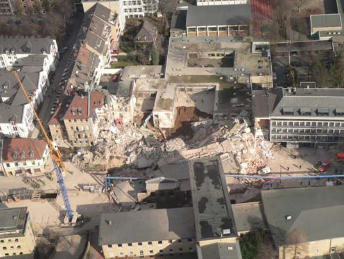
Figure 4. Aerial view of collapsed Historical Archive.
