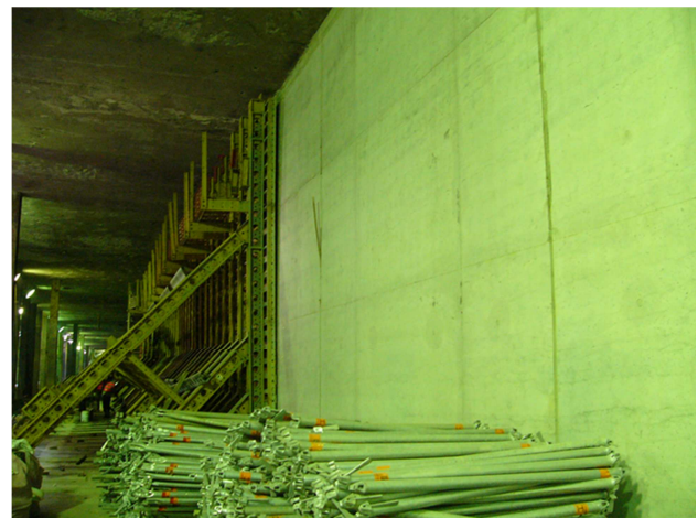
Photo-1 SCC concrete in B2F wall
