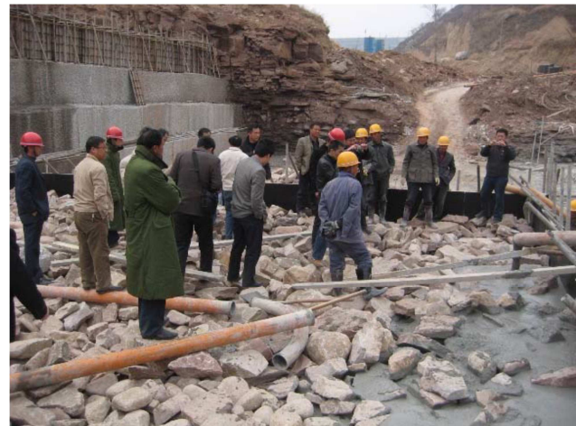
Photo-2 RFC construction
