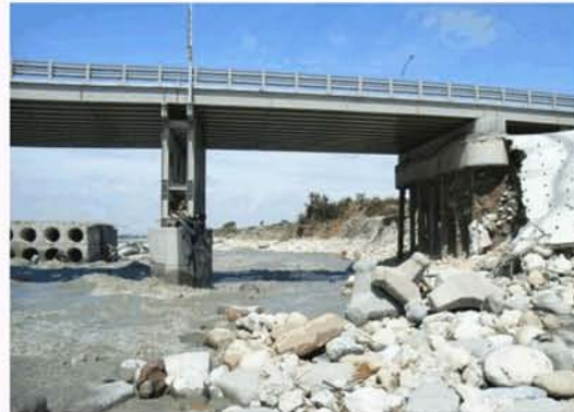
Photo 5.2 Temporary steel bridge with H-section steel pile
