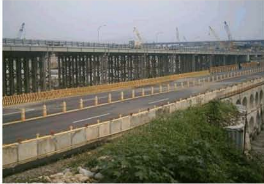
Photo 3.1 Completed temporary access bridge
