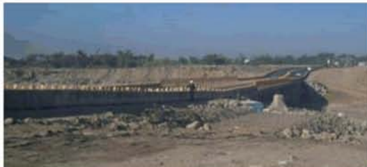
Photo 2.2 Completed temporary access road
