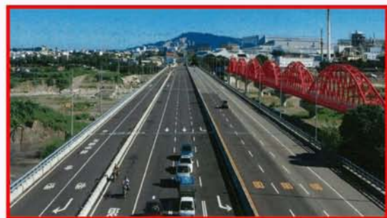
Photo 4.3 Completed Houfeng bridge
