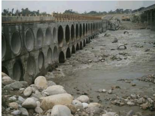
Photo 2.1 Temporary access road built by steel pipe and RCP pipe
