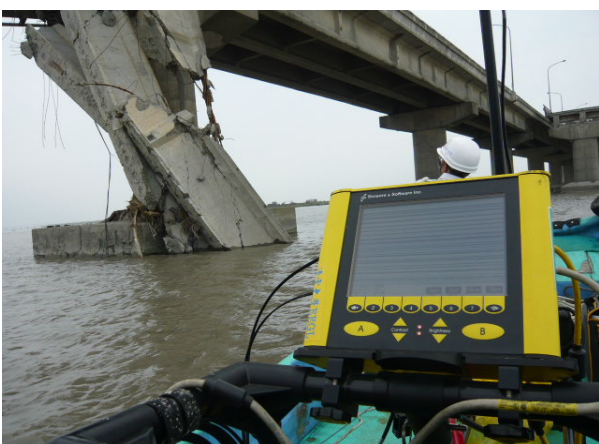
Figure 5 Underwater GPR and sonar inspection to Shuang-Yuan Bridge
