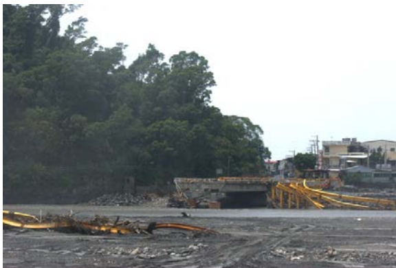
Figure 8 Severe debris flow destroyed Dajin temporary steel bridge
