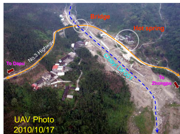
Fig. 6 UAV photo of Chiayi DF051 torrent after Typhoon Morakot
