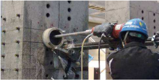
Figure-6 Actual situation (core drilling)
