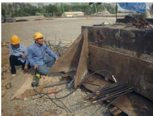
Fig.5.2.4: Tensioning PC strands
