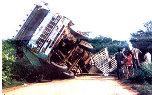
Fig.2.1.3.2 Overloaded truck caused the collapse of a bridge in Mongkul Borei on 07 Sep. 2004
