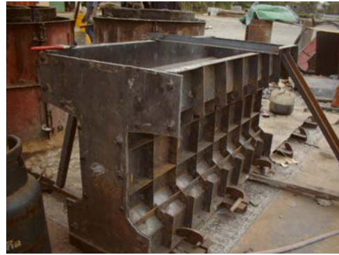
Fig.5.2.2: Formwork
