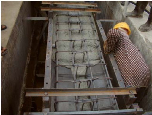
Fig.5.2.6: Casting SCC
