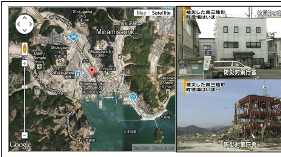
Figure 2.20 Minamisanriku Disaster Management Office before and after 2011 Tohoku Tsunami (Source: Minamisanriku City)
