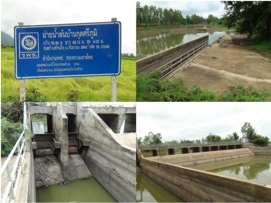
Figure 17 Kud Sri Phum weir project
