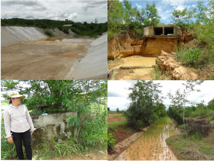
Figure 18 Wang Ta Ke project
