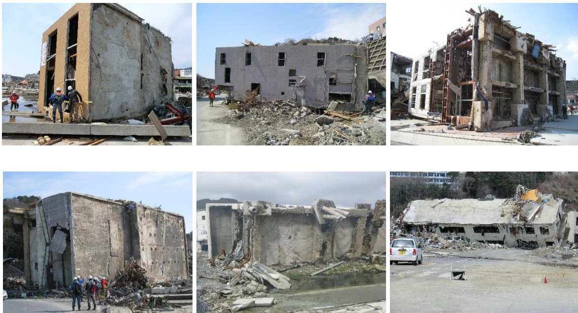
Fig. 1.5 Six overturned buildings in Onagawa town
