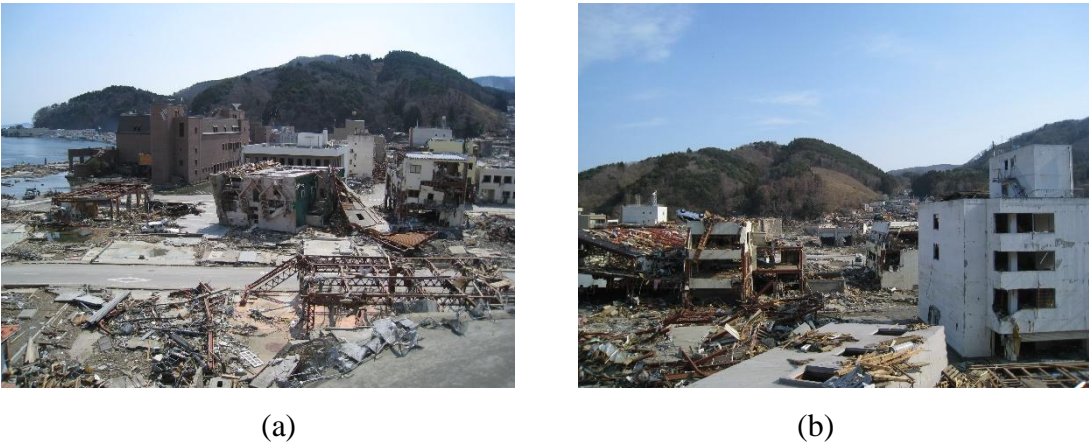
Fig. 1.1 Overall damage from earthquake and tsunami
