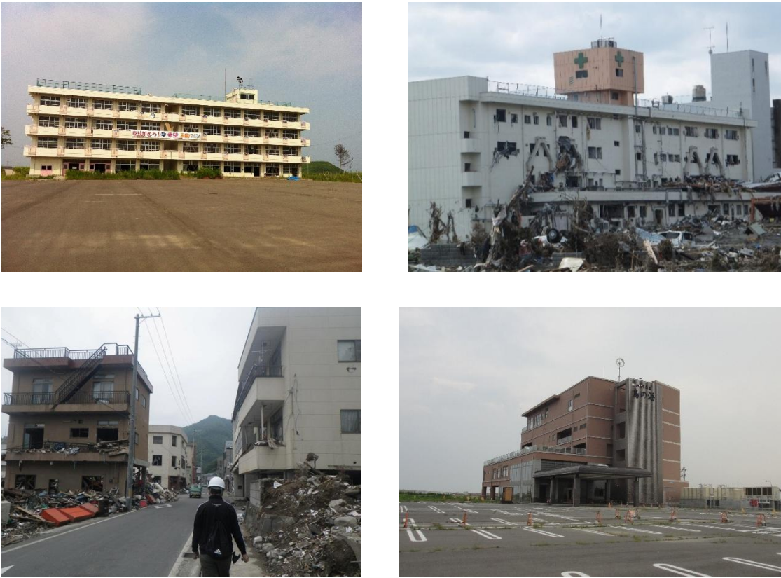
Fig. 1.4 Importance of RC building during earthquake and tsunami
