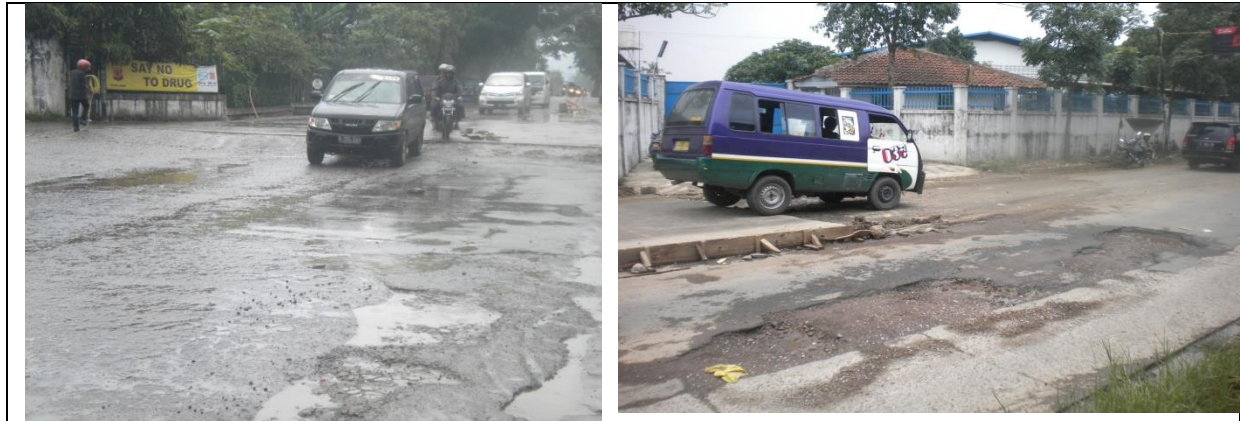
Figure 8 Poor Connection between old and new pavement in MM street
