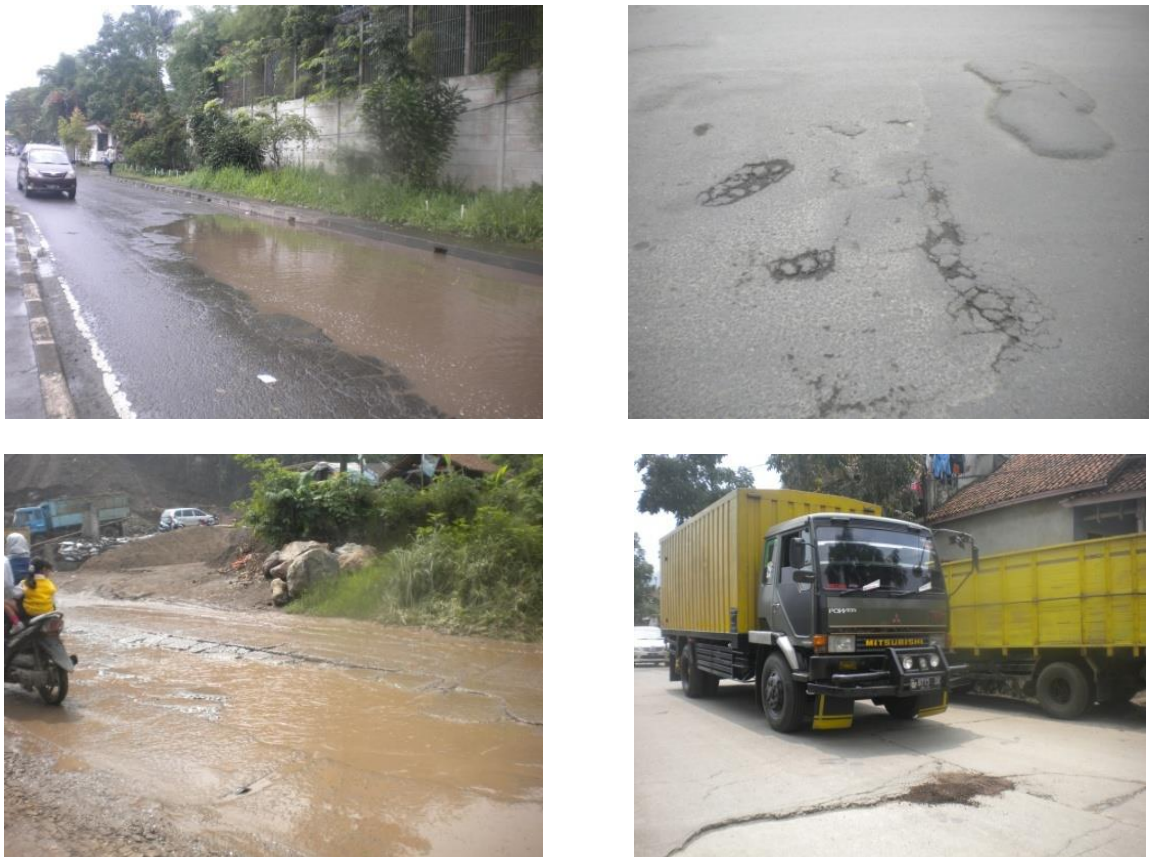
Figure 4 (Left) Water pond in MM and K street (Right) Pavement distress in MM andK street
