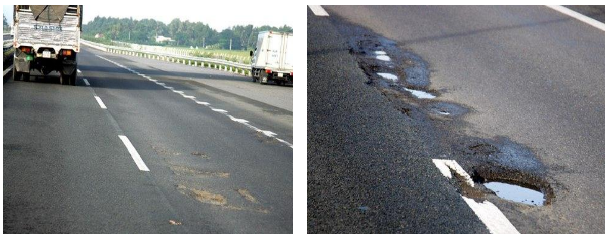
Figure 2.7 HCMC-Trung Luong express way' pavement with potholes and delves (source:Vnexpress News)
