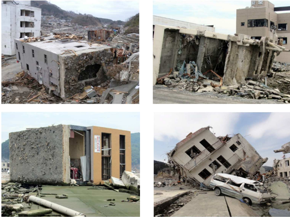
Figure I.3 Overturned buildings in Onagawa town [5]
