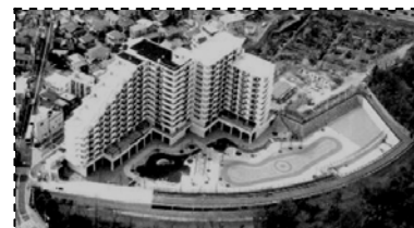
Fig.-2 Typical On-site Rainwater Storage Pond in Tokyo
