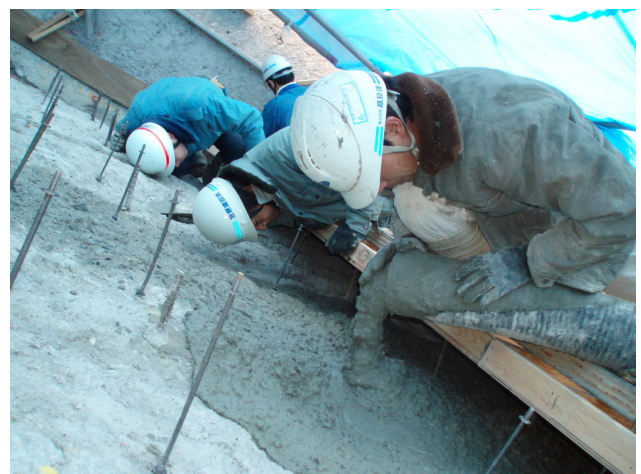
Photo-6 Placing of S.Q.C.
