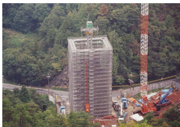
Photo-2 Concrete Placing
