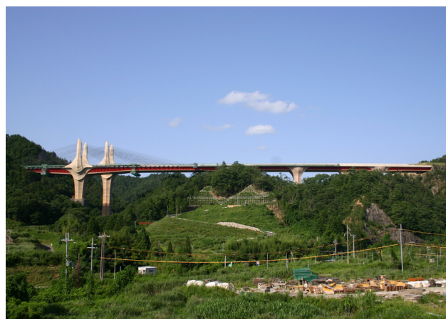
Photo-1 Ritto Bridge
