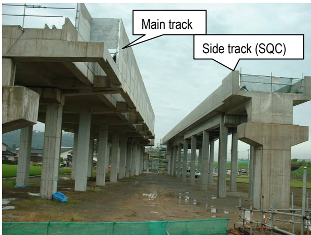
Photo-3 Viaduct of Kurobe maintenance base
