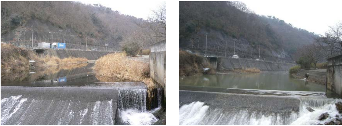
Photo 3. Excavation and Removal of Sediment Etc. at the Old Weir Upstream from the Reservoir (Fig. 1 Point B) (Left: before excavation, right: after excavation)
