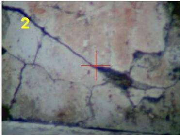
Figure 13 Crack target 2 measured by the image total station.
