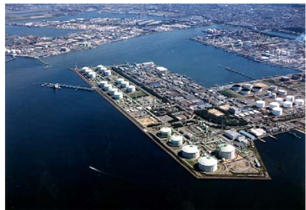
Figure 2 View of Senboku Terminal 2
