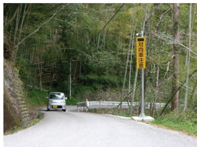
Fig5 Simplified type (fixed display board + LED)
