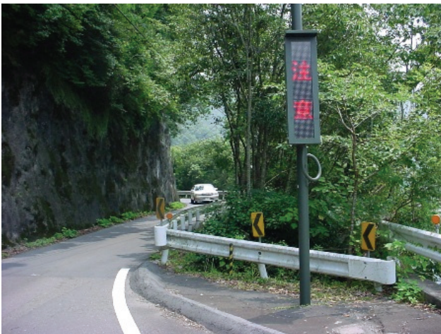
Fig1 Oncoming car approach indication system
