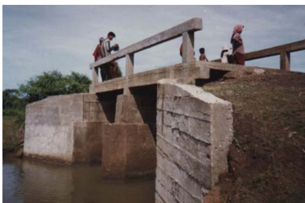
Fig.3 Reinforced concrete bridge
