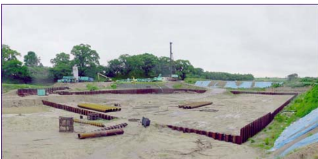
Figure 14 Construction Yard in Dry Condition
