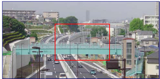
Figure 18 Tokyo Circular Road No.8 (red box: A Concrete Wall for Tokyo Circular Road No.8)
