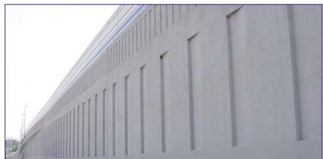
Figure 20 Whole View of the Concrete Wall
