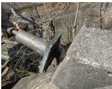
Picture 2. Degradation in anchor
