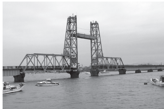
Photo 1.1 Chikugogawa Movable Lift Bridge
