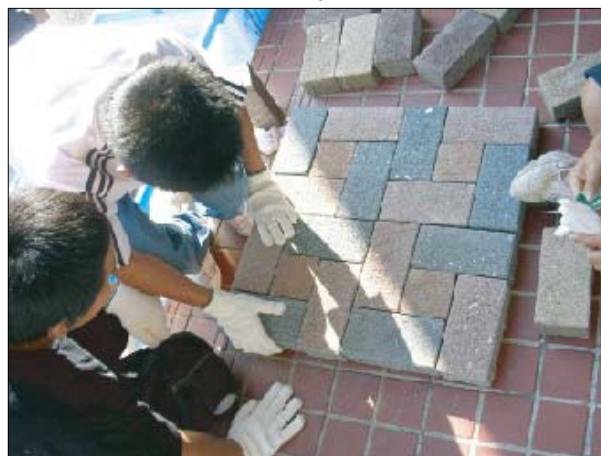
Photo 7 Decided combination of block
