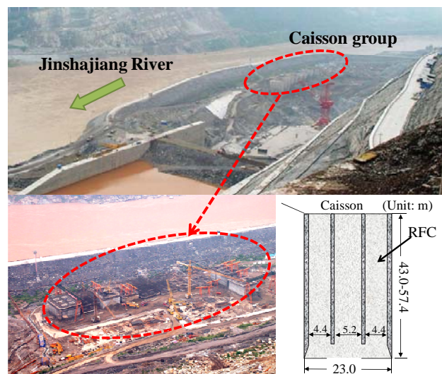
Figure 9 the Chinese biggest caisson group in the Xiangjiaba project
