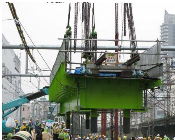
Figure 5 Scene of rail switchover (2)
