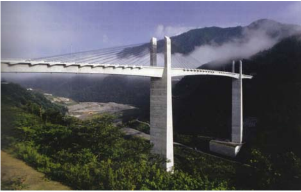
Fig.4 Extradosed bridge, Tokunoyama-Hattoku bridge, 220m, (Japan water agency and Oriental)
