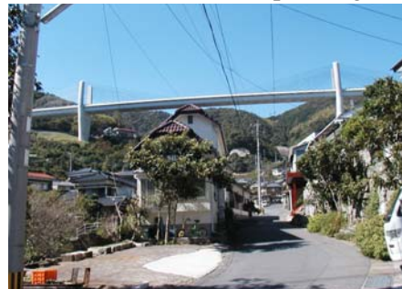
Fig.7 Extradosed bridge with corrugated steel webs, first completed, Himi-Yume bridge, 180m, (JH and Sumitomo)
