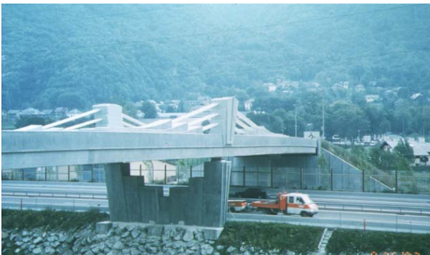
Fig.5 Another type of extradosed bridge, St Remy de Maurienne bridge, France
