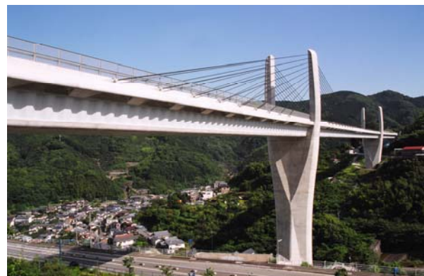
Fig.1 A Typical Innovative Bridge, Himi-Yume Bridge (Nagasaki Prefecture), JH and Mitsui-Sumitomo, Photo by courtesy of Mashiko
