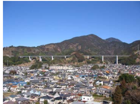
Fig.10 Steel truss webs, Saruta-gawa and Tomoe-gawa bridge, first expressway bridge, (JH and Ohbayashi)
