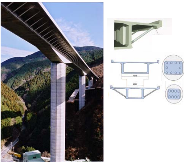
Fig.12 Strut supported slab of the bridge with very high piers, Shibakawa viaduct, (JH and Oriental)
