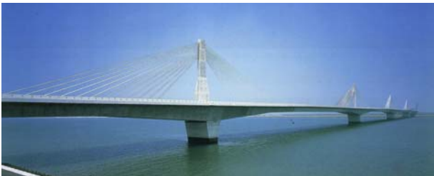
Fig.2 Extradosed bridge, Kiso-gawa and Ibi-gawa bridge, 275m (JH)
