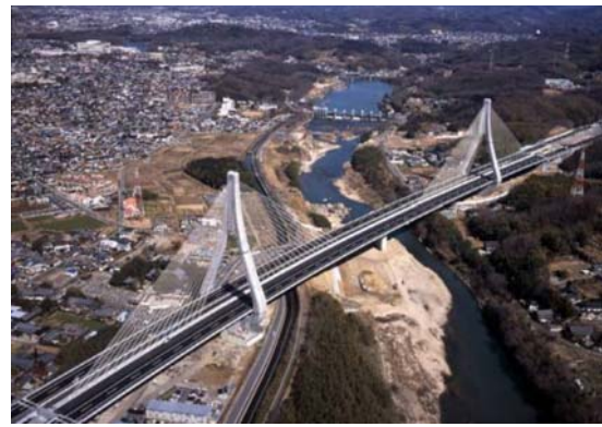
Fig.9 Cable stayed bridge with corrugated steel webs, Yahagi-gawa bridge, (JH)
