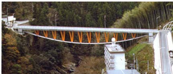
Fig.15 Suspension cable supporting roads above, construction bottom up, Seiun Bridge, (Tokushima prefecture and Sumitomo)
