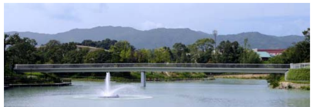
Fig.18 Slender and straight profile of beam by UHPC, Mikane-ike foot bridge, (Ohnojou city, Fukuoka prefecture and Taisei)
