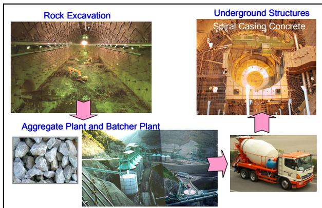
**Fig.4.7 Recycle of Excavated Rock**
