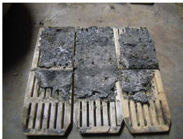
Picture 3. Clinker adhered to the ceramic rostile
