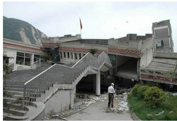
Fig. 9 The collapsed RC school building
