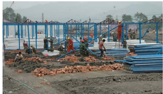
Fig. 42 The temporary houses under construction near Pongzhou.
