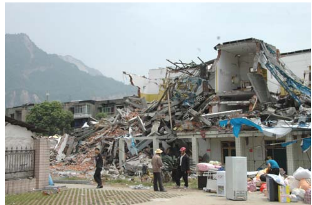
Fig. 11 The collapsed dormitory of a hospital
