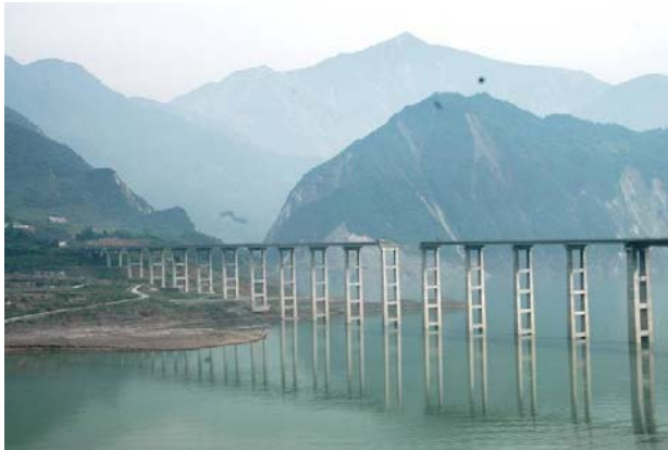
Fig. 28 The falling span of Miaotzuping bridge
