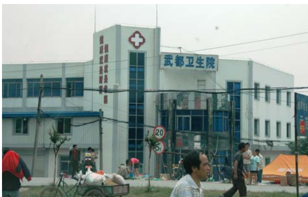
Fig. 14 The hospital is out of service
