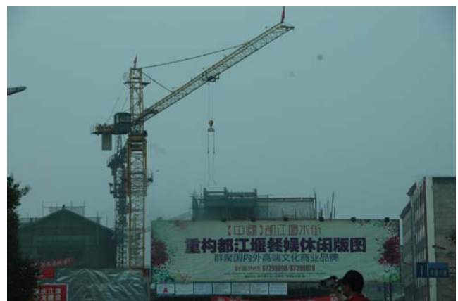
Fig. 22 The crane tower is still in operation
