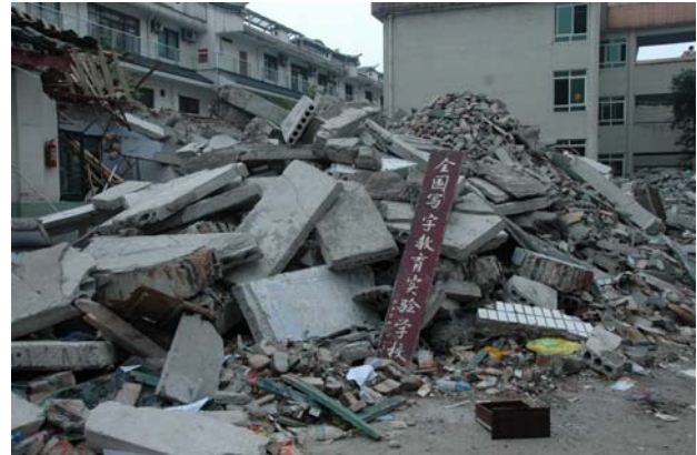
Fig. 3 The collapsed URM building in school
