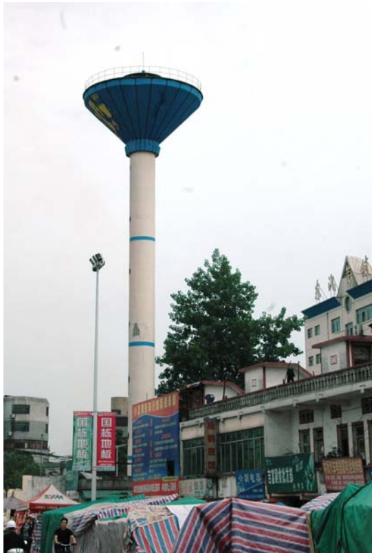
Fig. 19 The water tower is still standing
