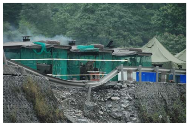
Fig. 36 The China army is guarding the damaged bridge
