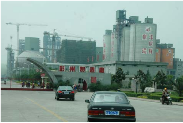
Fig. 18 The concrete pre-mix factory was intact
