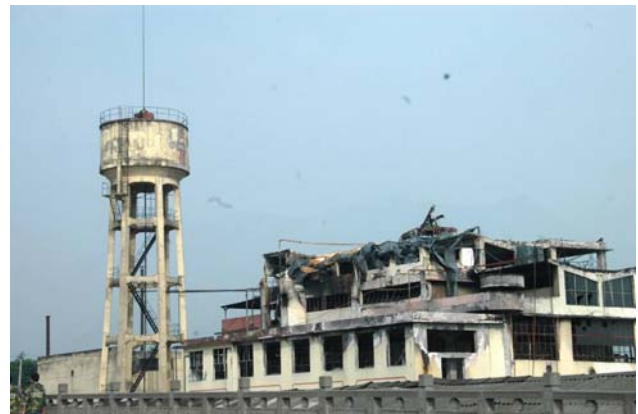
Fig. 21 Another undamaged water tower
