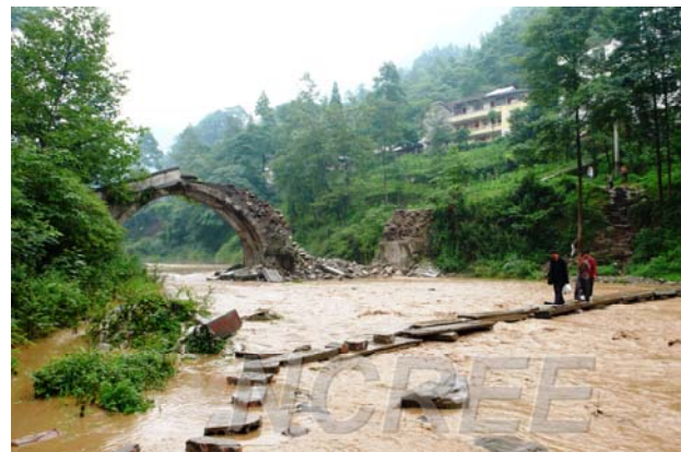
Fig. 29 The destroyed arch bridge in Bailu
