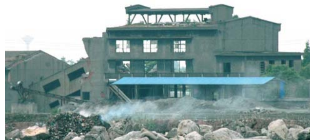
Fig. 16 The collapsed factory
