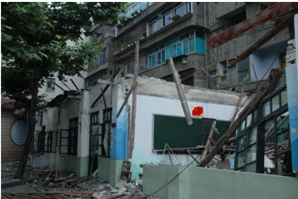
Fig. 2 The collapsed masonry classrooms
